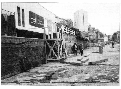
Paddington Basin is currently de-watered to be cleared of silt and have some changes made to the waterway wall in connection with development around the site.
